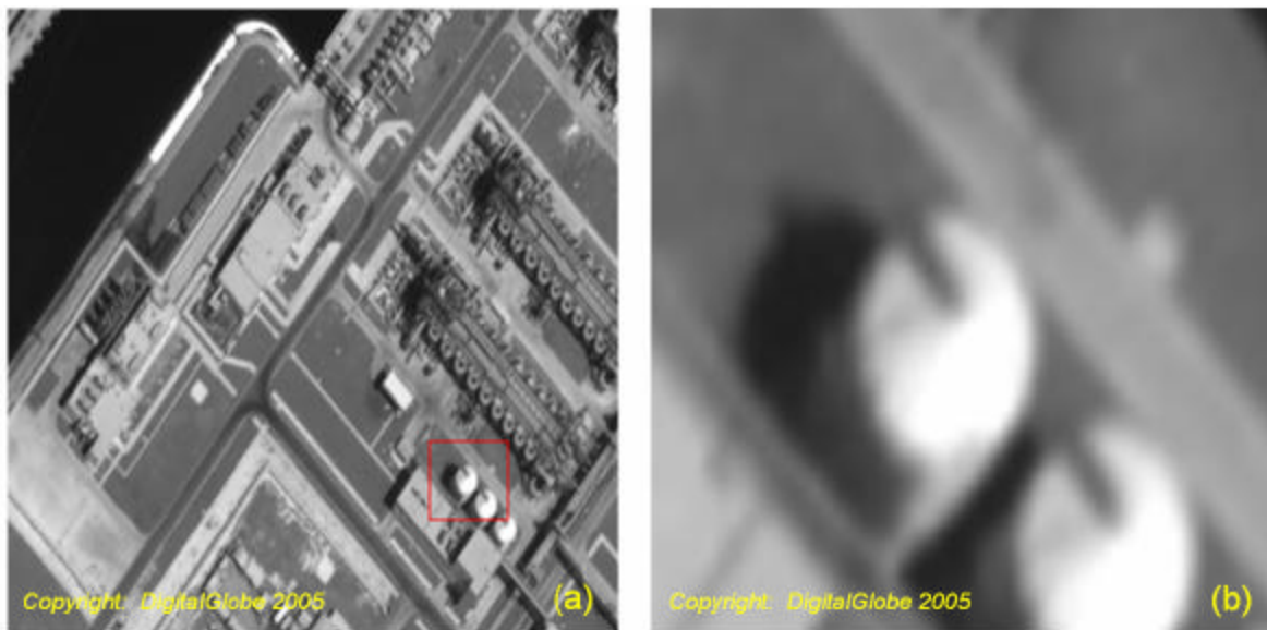
Figure 1. An example subset of a QuickBird panchromatic image of a water desalination plant northwest of Abu Dhabi taken 26 September 2004: (a) general overview of the area and (b) a zoom showing and individual shadowed area (courtesy of DigitalGlobe).
